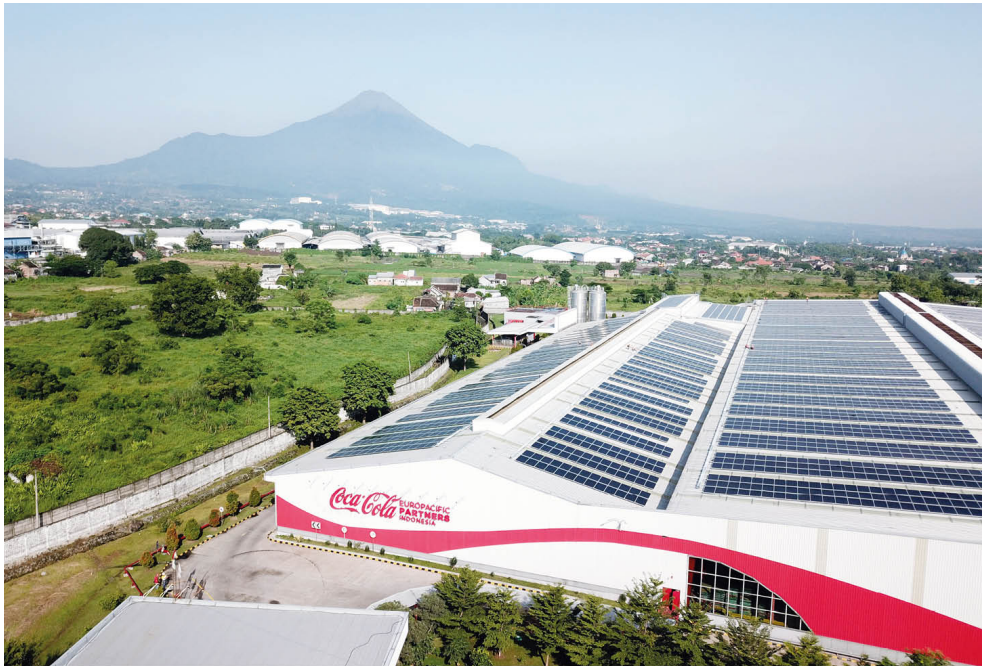
Above: Solar panel installation at our production facility in Cibitung, Indonesia
